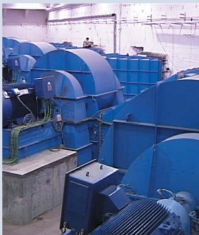
Centrifugal ventilation fans being installed at the Mont Blanc Tunnel.
