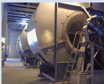
Howden Buffalo centrifugal ventilation fans supplied to the Boston Central Artery Tunnel.
