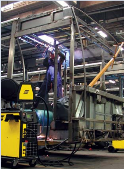
Welding of stainless steel bus frames at Van Hool bus and trailer plant in Belgium
