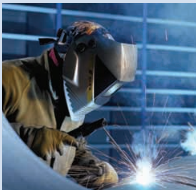
Manual welding of pipelines using ESAB manual electrodes
